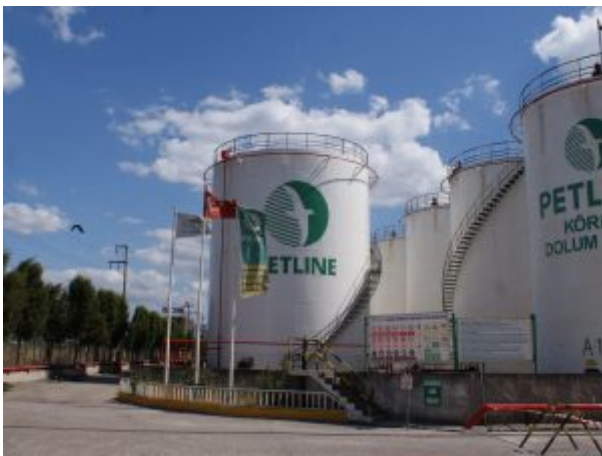
Petline pretrol filling station
