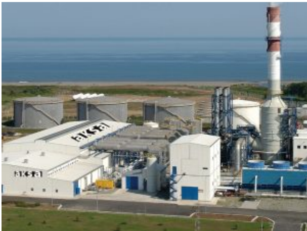
mobile power plant
