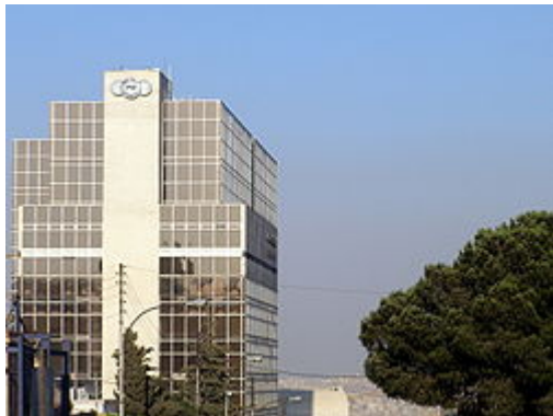
Arab bank headquarters building
