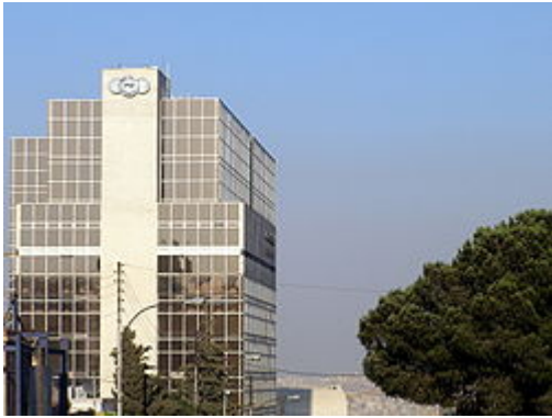
Arab bank headquarters building
