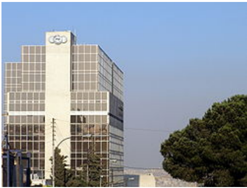
Arab bank headquarters building
